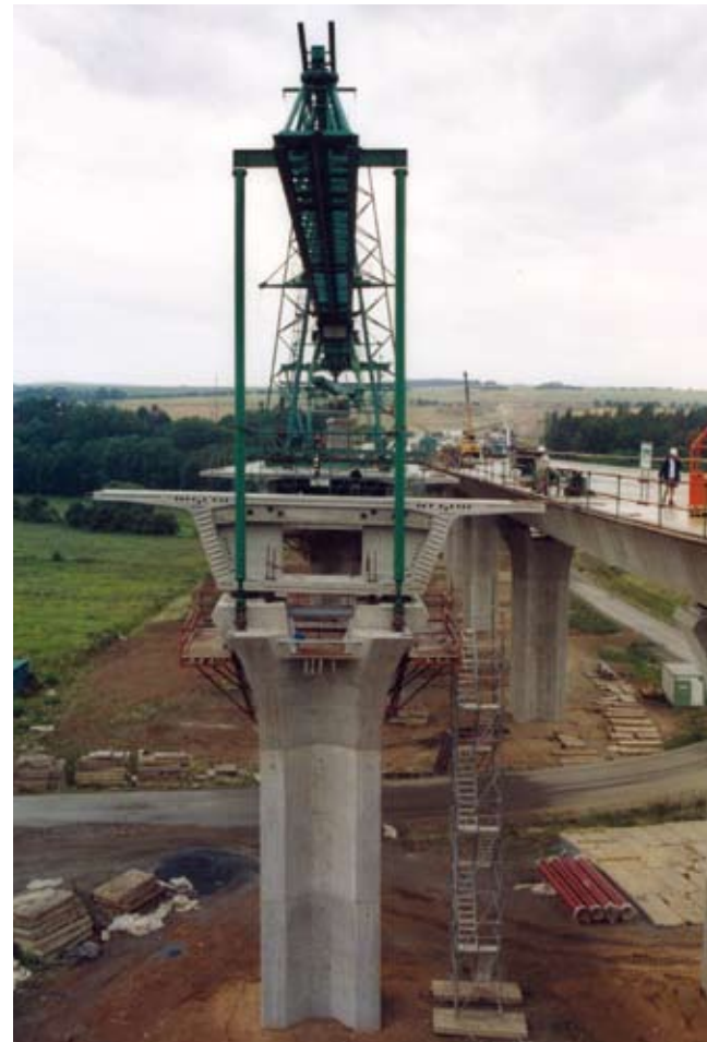
Uhlavu Bridge, Pilsen, Czech Republic
