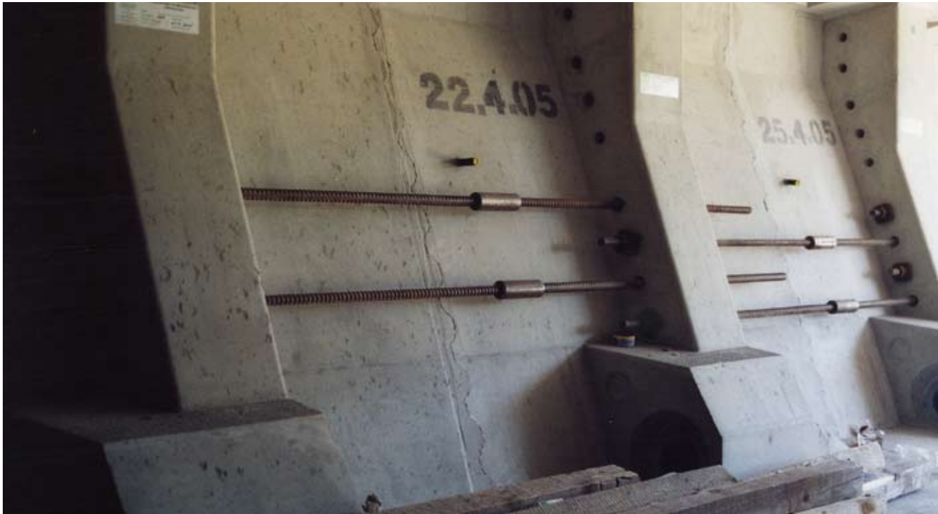
Typical Coupling, Uhlavu Bridge, Pilsen, Czech Republic
