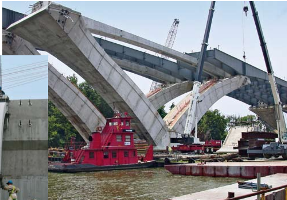
Woodrow Wilson Bridge, Washington, D.C., USA
